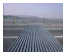
Modular expansion joints
