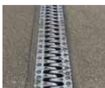
Cantilever finger joint
