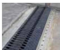
Sliding finger joints
